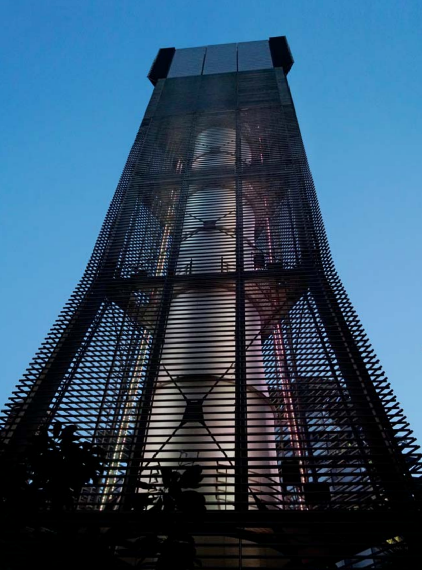
Left: A 45-meter high harvester of the wind, Masdar City's tallest structure is a modern version of the region's traditional barjeel , or wind tower. Using a Teflon™-coated tube, it channels breezes to ground level. Right: Professor Alexander Slocum and Solar Platform Chair Nicolas Calvet flank their research colleagues at Masdar's prototype solar Beam Down Tower. It uses focused sunlight from 33 mirrors to melt a thermal energy storage reservoir of four tons of salt, which can be used to drive steam turbines both during the day and at night.
